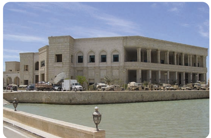
DataPath terminals and personnel rolled into Iraq in 2003 with U.S. forces and have worked side by side with them there, including at forward operating bases, ever since.
